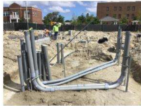
Electrical duct banks.
