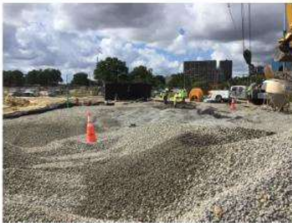
Back filling underground water retention system.
