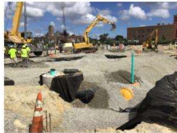
Backfill of underground storm retention system.
