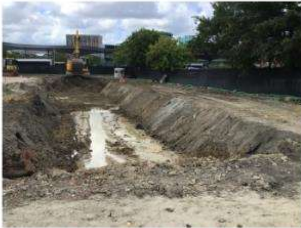
Excavation for underground retention system.
