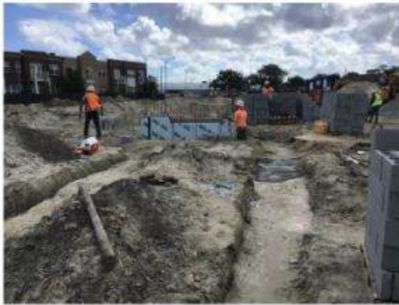
Footings in place, elevator shaft in progress.
